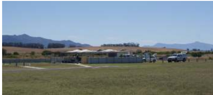
General view of the TMFC facilities.
