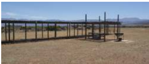
Covered pit area provides some shade.
